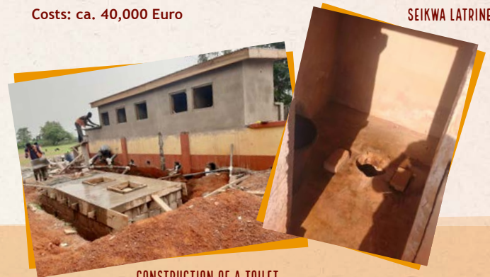
CONSTRUCTION OF A TOILET FACILITY – FINAL STAGES
