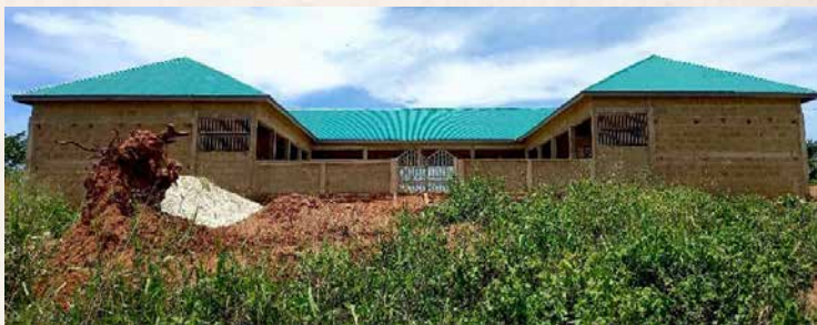
PRIMARY SCHOOL AMPAHA MAY 2021
