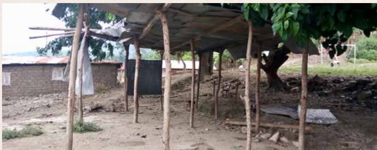
LAKESIDE ESSAASE KINDERGARTEN BEFORE
