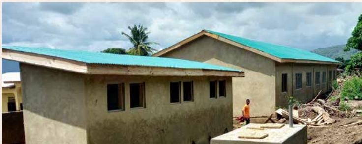
LAKESIDE ESSAASE KINDERGARTEN AND TOILET FACILITY JUNE 2021
