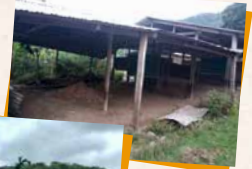
KINDERGARTEN ESSAASE LAKESIDE - BEFORE
